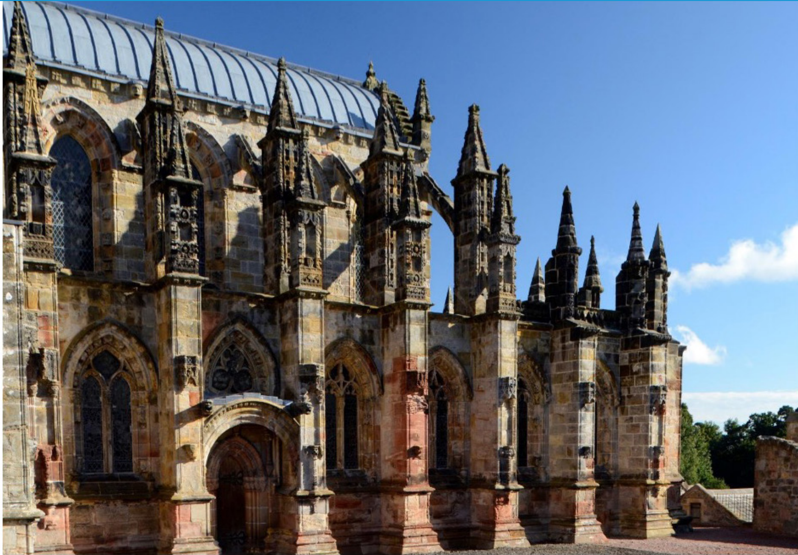
Flying buttresses and pinnacles
